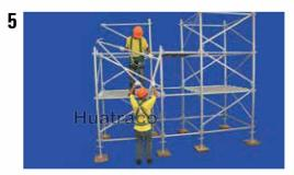
Erection must be carried out from the inside of towers. Fit the triangle at lift 3, provided complying with the safety regulations protected by the triangle of the lower lift. The temporary platforms from lift 1 are moved to lift 2.
