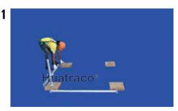
Position the jack bases at the intervals determined by the ledgers. Fit the basis standards into the jack bases. Then fit the first plan braces, rings downwards.
