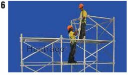
Fit triangle at lift 4 and erect safely from second platform. Reverse the direction of the triangle.
