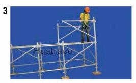
Fit the second lift of the triangle, reverse the direction of triangle.
