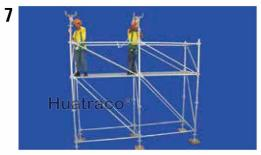
Clamp the 3<sup>rd</sup> level of ledgers, fix the diagonal braces and insert the U-heads.
