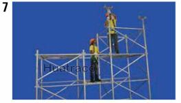
Link up the standard with the ledgers. Insert the U-heads into the vertical posts/standards.
