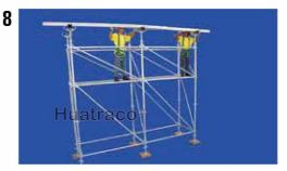
Place the primary & secondary of soffit formwork and secure plywood / panels on the secondary.
