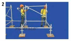
Clamp the 1st level of ledgers. Insert and lock the first lift of triangle. Check the structure is level.
