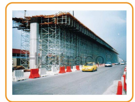
Huatraco® C60 Shoring System is a multi-directional & multi-level heavy duty shoring equipment to support all types of heavy structures, and is manufactured to comply with British Standard BS 5975 and BS EN 12812.
