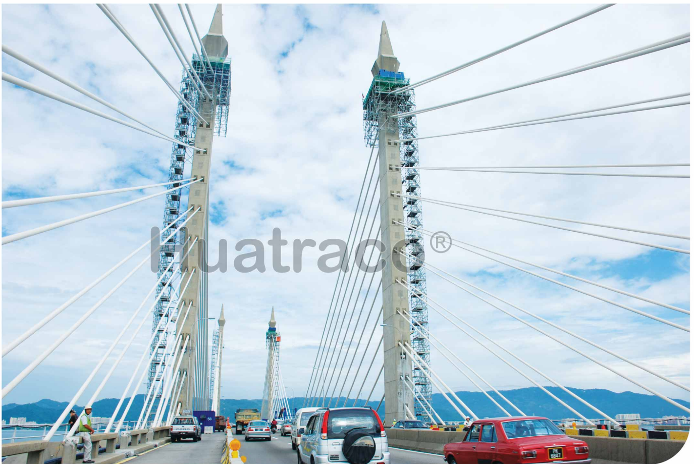
Pylon Access Tower, Penang Bridge, Malaysia
